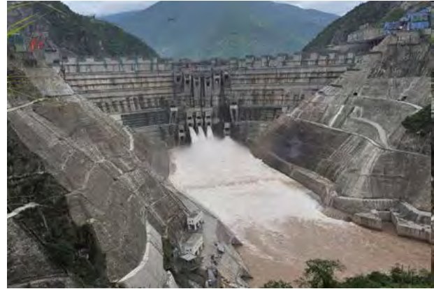
Figure A-3.5 Xiaowan Hydropower Project. (Source: Mekong River Commission)
