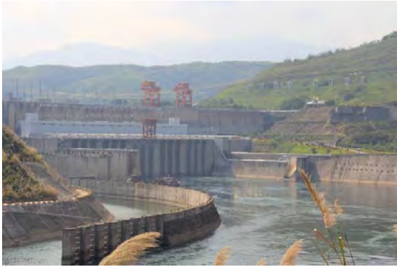
Figure A-3.1 Jinghong Dam (Source www.flickr.com )
