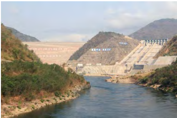
Figure A-3.2 Nuozhadu Hydropower Project (Source www.flickr.com )
