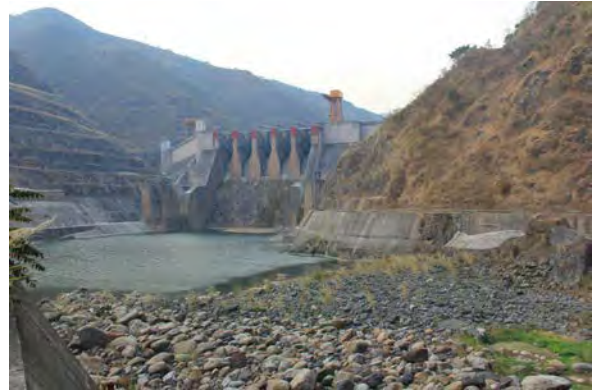
Figure A-3.3 Dachaoshan Hydropower Project (Source www.flickr.com )
