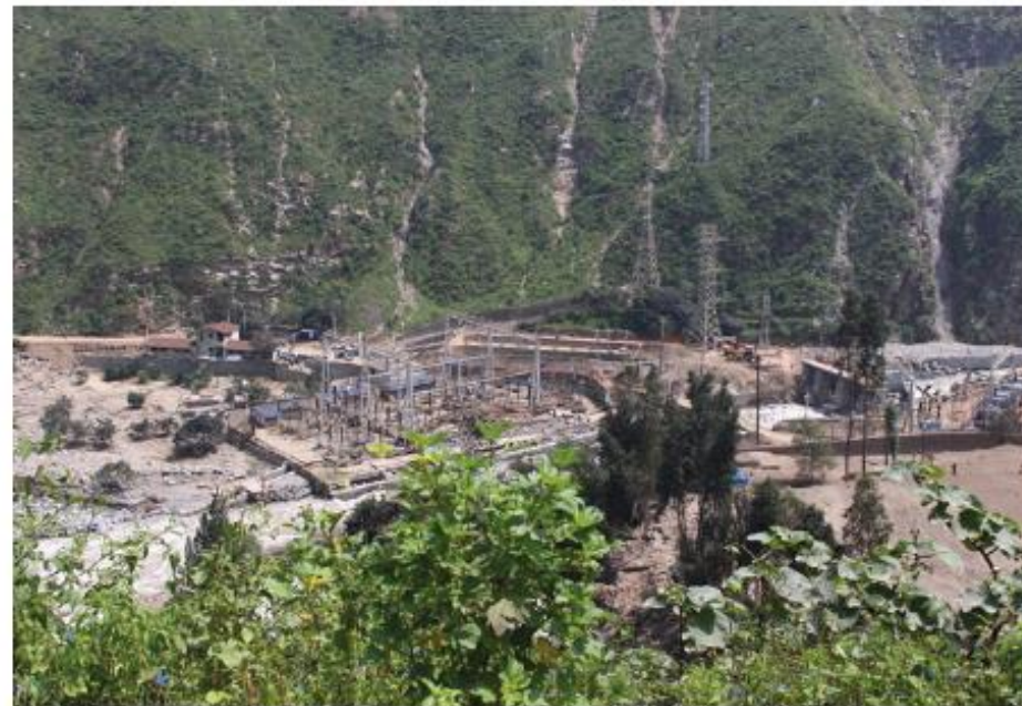
4.) Callahuanca's hydroelectrical power plant in Santa Eulalia's sub basin, after the flood disaster in March 2017
