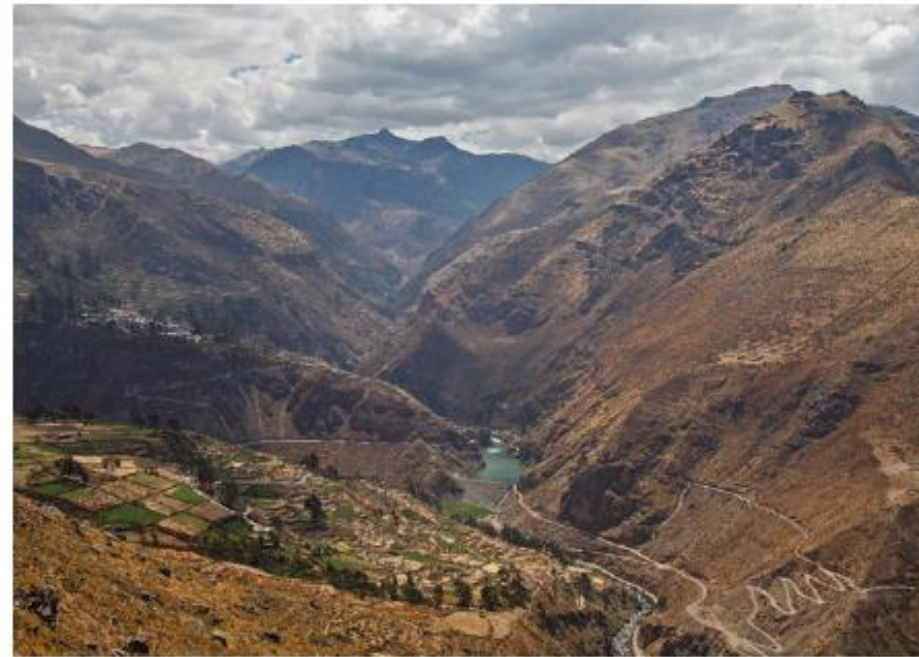
2.) Sheque dam, in the upper part of the Santa Eulalia's sub basin
