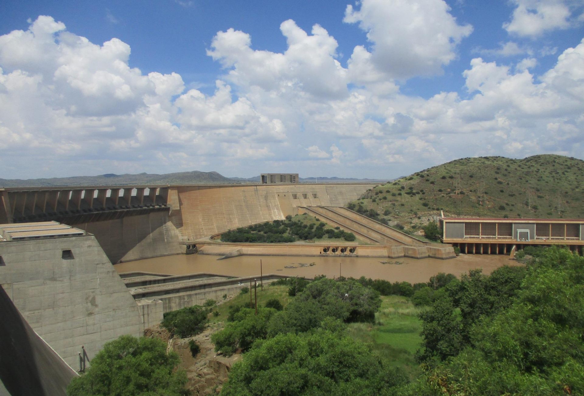
Gariep Dam, South Africa
