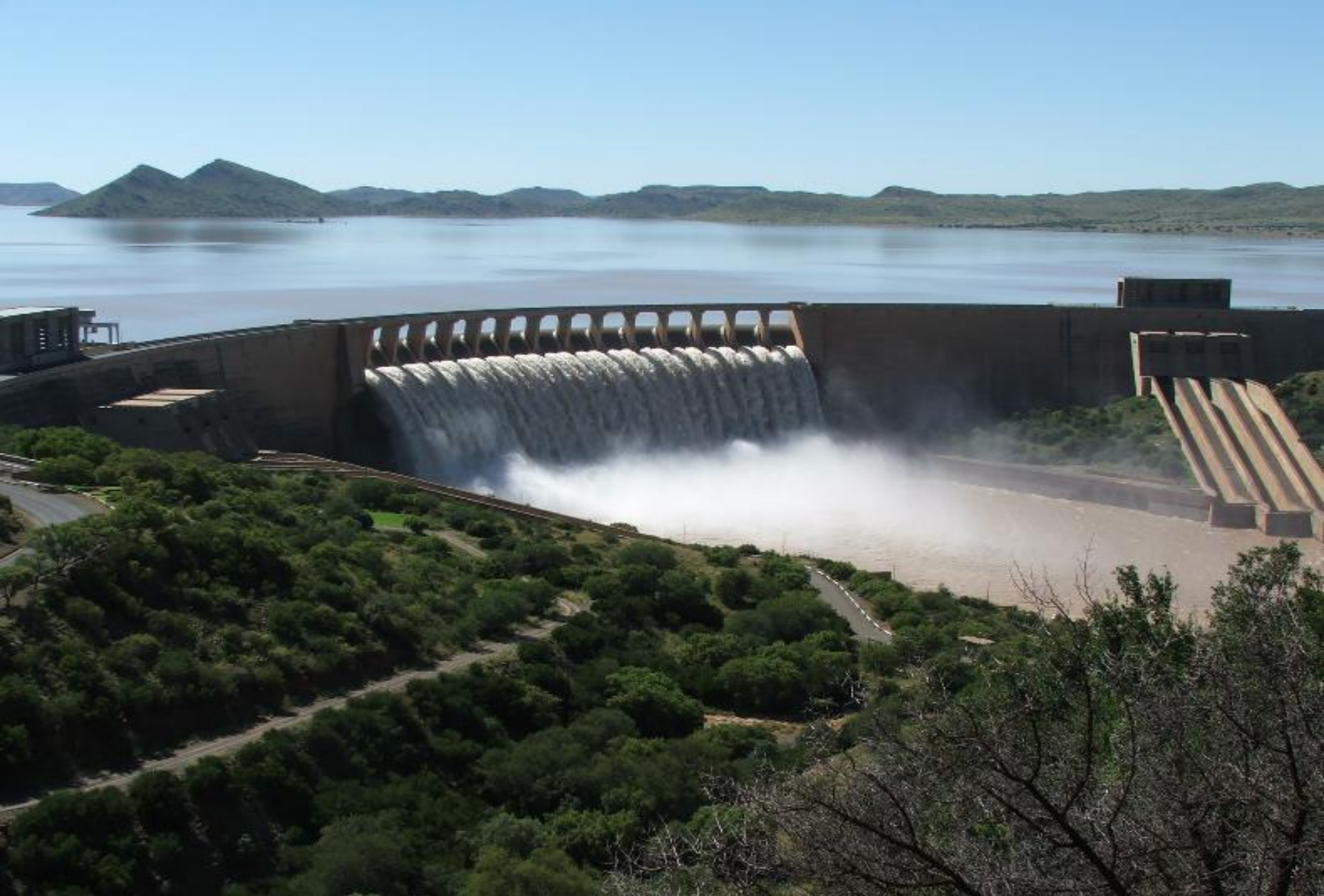
Gariep Dam, South Africa
