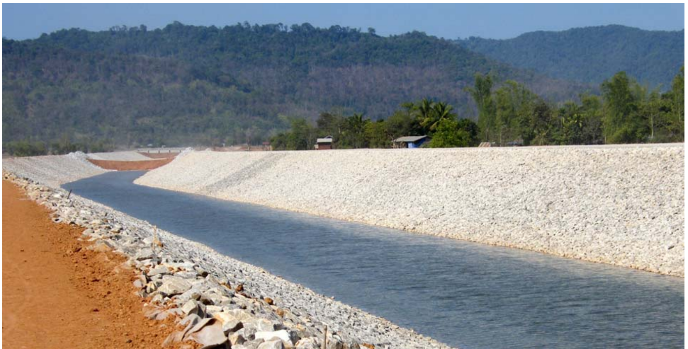
The downstream channel constructed below the power station takes 350 m 3 /s of turbinated water down to the Xe Bang Fai river, adding significantly to its normal background flows and seriously impacting the aquatic ecology and river-dependent livelihoods (Source: Aurecon Group)
