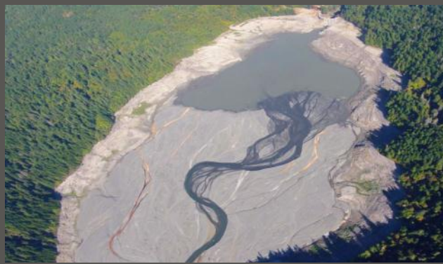
Over flooding and storage capacity reduction
