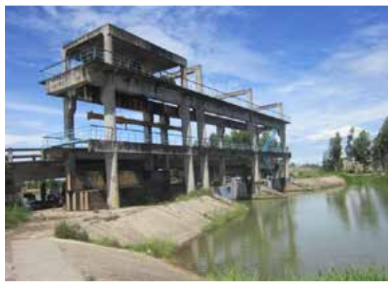
Figure 4: Sluice for saltwater control in VMD
